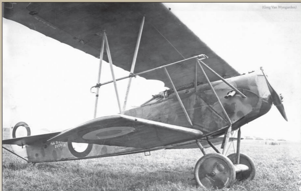
Fokker D.VII (OAW) 2009/18 was the first D.VII captured intact and as such was extensively evaluated by the French and then the British. OAW style component stencils can be seen on the aileron, wheel cover, wing 'N' strut and rear 'cabane' strut. Some early production identifying features are the smooth cowlings with 'organic' pattern camouflage, white datum line and the serial number painted in white at the rear of the fuselage. The large pitot fitting attached to the wing was added during the post capture evaluation by the French.
