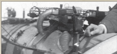
Cockpit coaming and LMG 08/15 'Spandau' detail from E . Note the small windscreen C2 , padding and empty belt chutes A12 & A13 .
